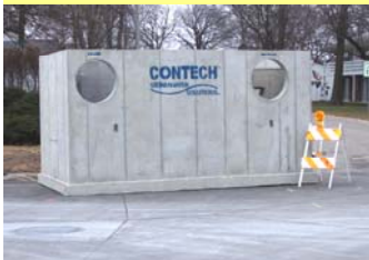
Grit collection chamber prior to installation at Bayside Ave. boat ramp.
