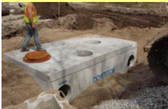
Grit collection chamber being installed at Clear Lake.
