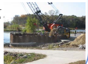
Construction of new outlet structure for Ventura Marsh
