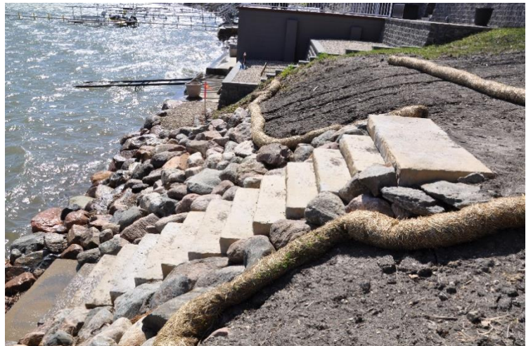
Photos (left) show the bank prior to restoration at the Hill Street public access dock in Oakwood Park, where the steep slope was covered by shallow-rooted non-desirable vegetation. The photo (right) shows the project currently underway, where the toe of the slope was stabilized with rock to minimize shoreline erosion, stone steps provide new access to the lake, and where the upland portions of the shoreline will be restored to prairie.
