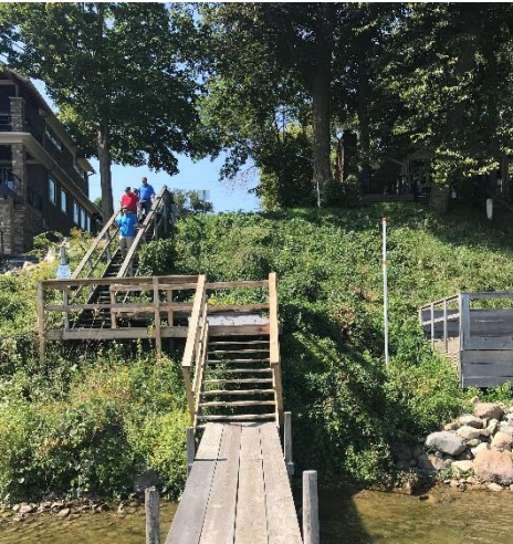
Photos (left) show the bank prior to restoration at the Hill Street public access dock in Oakwood Park, where the steep slope was covered by shallow-rooted non-desirable vegetation. The photo (right) shows the project currently underway, where the toe of the slope was stabilized with rock to minimize shoreline erosion, stone steps provide new access to the lake, and where the upland portions of the shoreline will be restored to prairie.
